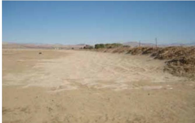
**Figure 14:** View (looking north) of 6 foot high frontline berm that borders the western edge of Rancho Seco, showing accumulation of captured sand on the upwind face of the berm.
