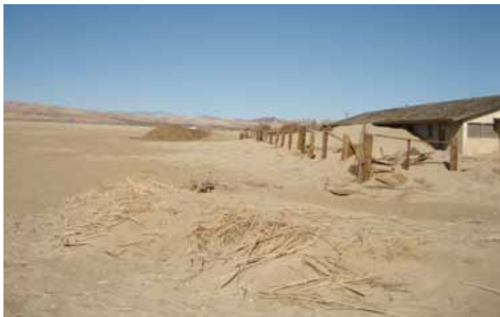
Figure 4: Sand deposits on the windward side of this house make it uninhabitable.
