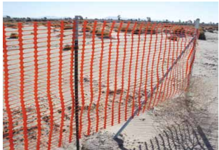
Figure 7: This 50% wind porosity fencing causes dust to deposit more on the downwind side of the fence.
