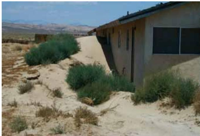
**Figure 13:** Rancho Seco residence has sand accumulation on the upwind side of the house.
